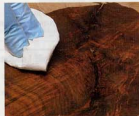
Scrape and sand until the surface is smooth and level. After the cyanoacrylate glue has dried, sand to a smooth finish. Wipe with a solvent to check the fit of the repair.
