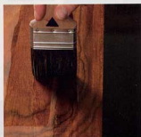
Blend the lines together. The tip-off stroke fills the gap, creating a finish of uniform thickness.
